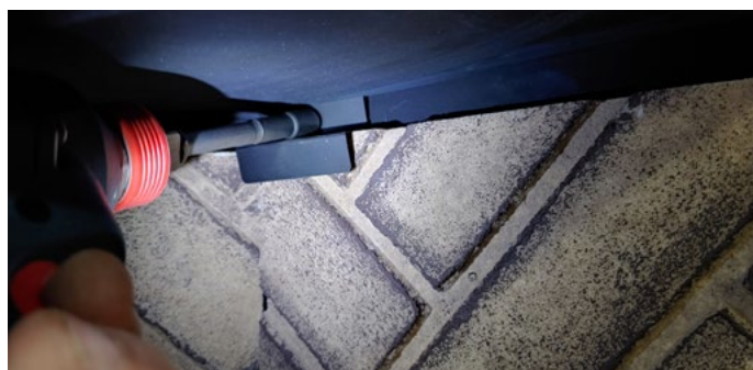
Figure 20.b Secure with the bracket using screw
