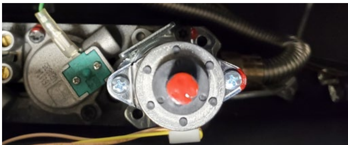
Figure 13.eee LP pressure regulator on a Full Load
