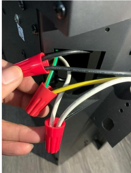
4. Return the cover plate to the left side, adding a wiring protector which you can find in the manual bag, and screw the two screws back in to fasten the plate.
