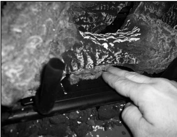
Figure 14.24 Placement of Rockwool Under Front Logs
