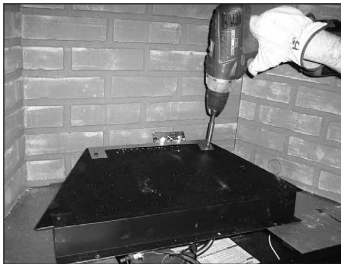
Figure 14.29 Remove Screws Attaching Back Burner Support
