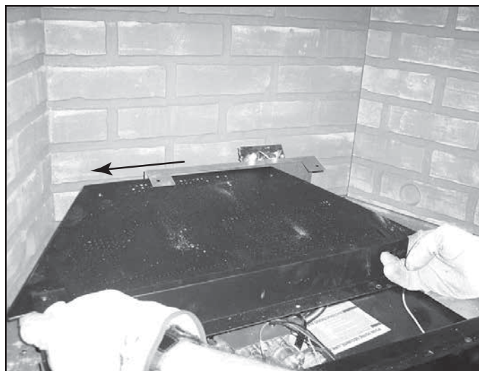
Figure 14.30 Side Burner Assembly to Left
