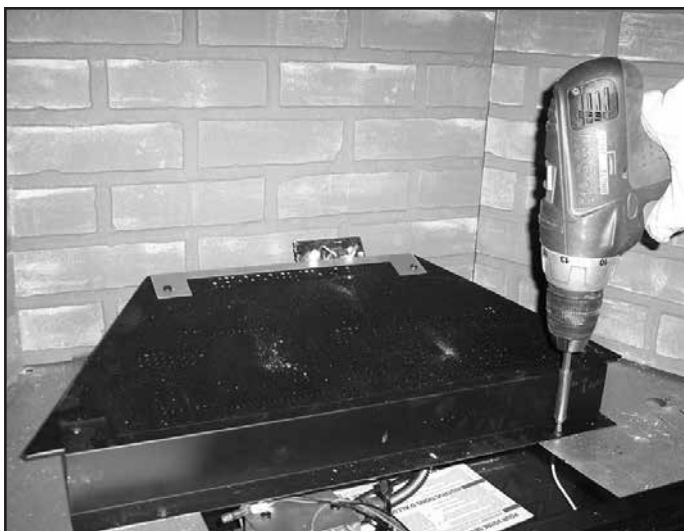
Figure 14.28 Remove Screws Attaching Front Burner Support
