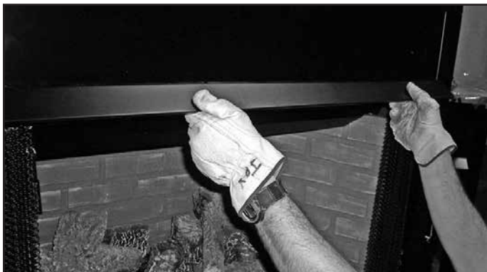
Figure 14.27 Installing the Hood
