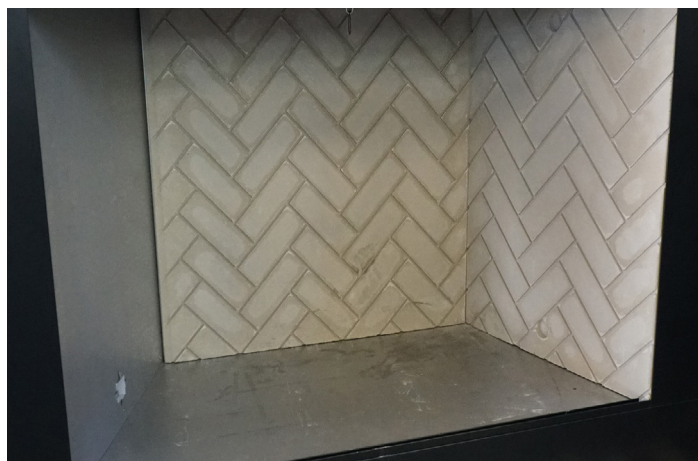
Install Right Side Refractory Brick Liner Figure 50
