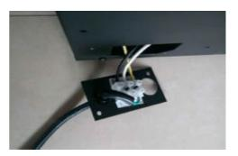
2. Attach the wiring to the junction block. Please make sure the live wire goes into the "L", the neutral wire into "N" and the ground wire into "G".
