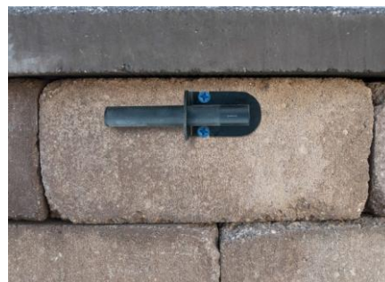
Figure 6.5 – Fasten down the bracket
