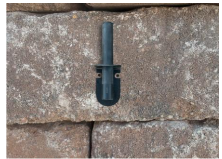
Figure 6.8 – Dry fit the bracket
