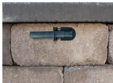
Figure 6.4 – Dry fit the bracket
