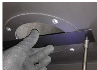
Figure 8.b.c Restrictor plate Installation
