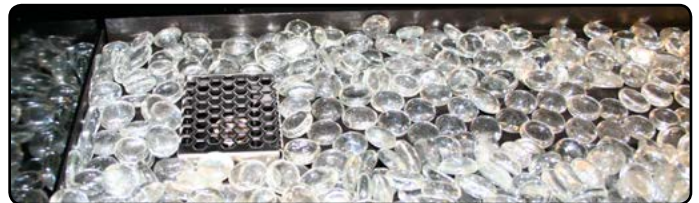
Figure 24.b Completed firestone installation
