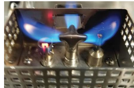
Figure 10.2 – Pilot flame coverage of thermocouple.
