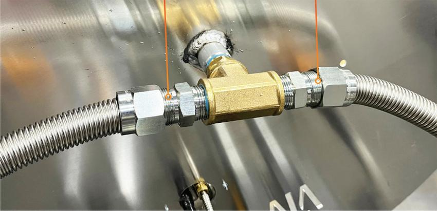
Photo 20: Connecting the Flex Lines
