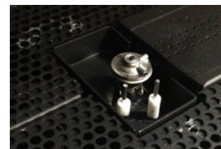
Figure 13. Removal of pilot cover
